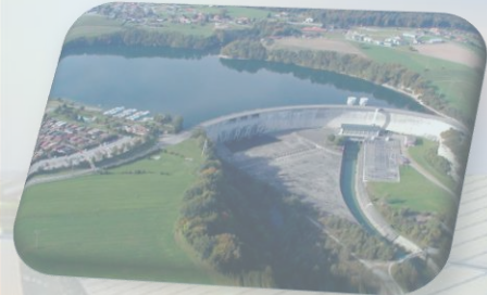
Schiffenen Dam in Fribourg, Western Switzerland. (Picture: Groupe E)
